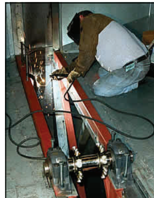
Structural Improvements at Cedars
