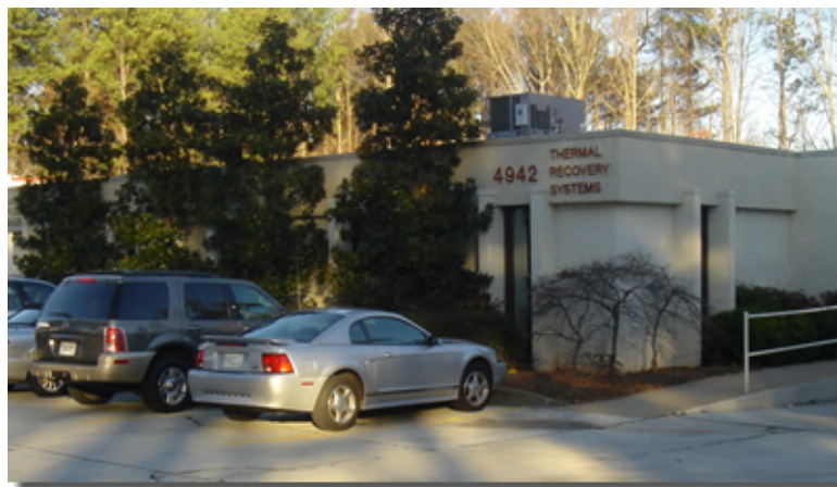
Thermal Recovery Systems Offices In Atlanta, Ga.
